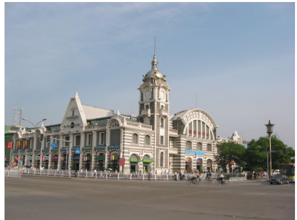
Railway Station Old 117-1799
