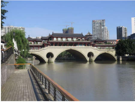
Chengdu #0655 Jinyang River Bridge
