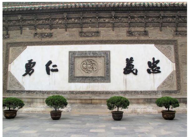
Shan Shaan Gan Clanhouse #6222 Screen Wall
