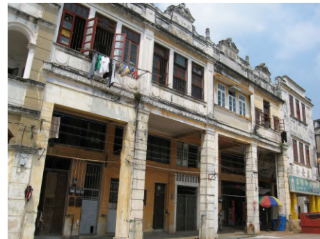
Kaiping #9074 Chikan Late Qing and Early Republic Buildings
