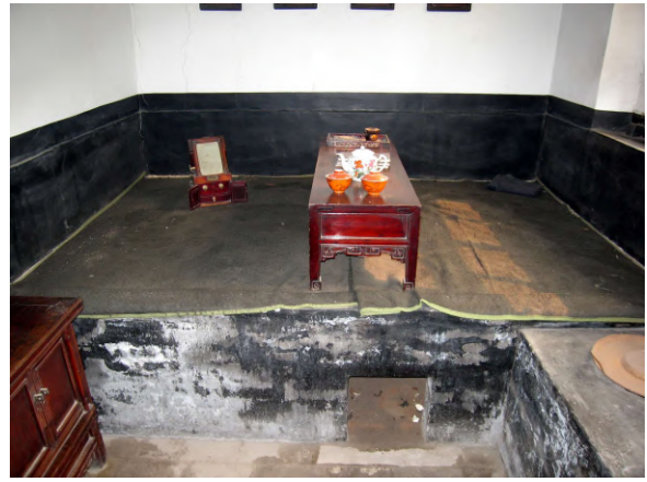
Wei Tai Hou Bank #2465 Bed with Heating Below
