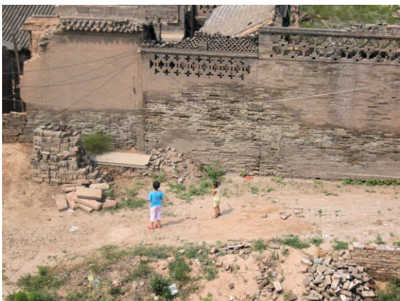
Walls #2127 View from Walls
