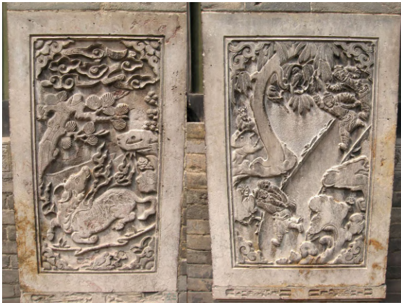
Wang Family Compound #2855 Decorative Stonework
