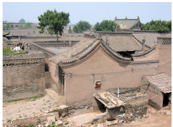
Walls #2128 View from Walls
