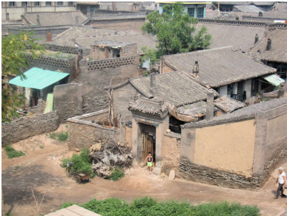
Walls #2134 View from Walls
