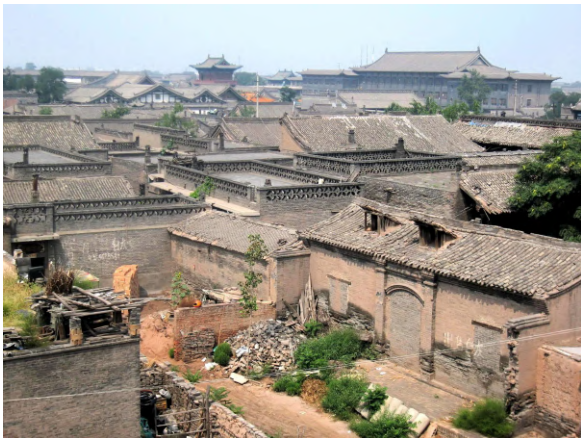
Walls #2149 View from Walls
