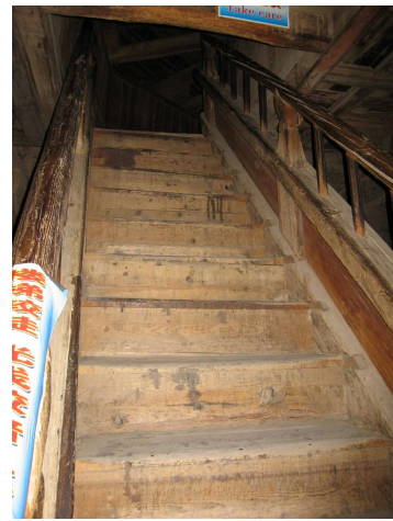
Yingxian Wooden Pagoda #3872 Built 1056 AD, Interior
