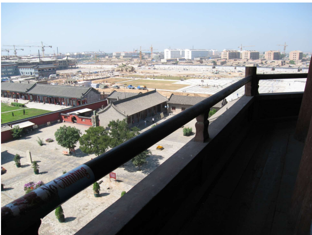
Yingxian Wooden Pagoda #3879 Built 1056 AD, View
