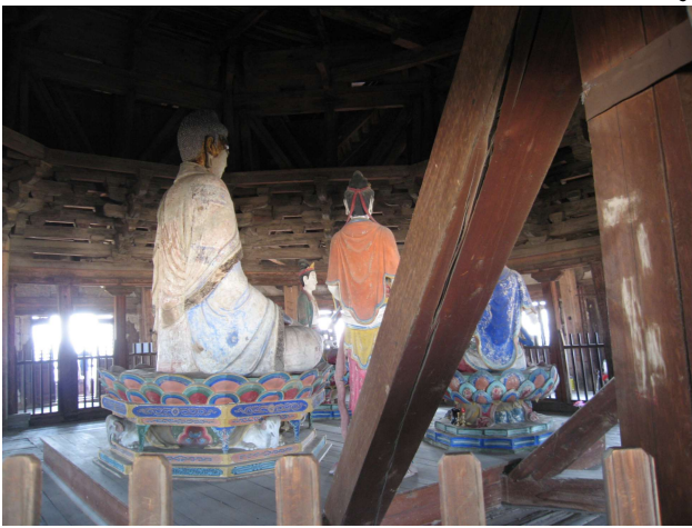
Yingxian Wooden Pagoda #3882 Built 1056 AD, Interior
