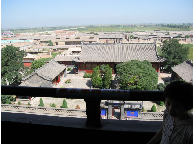
Yingxian Wooden Pagoda #3873 Built 1056 AD, View
