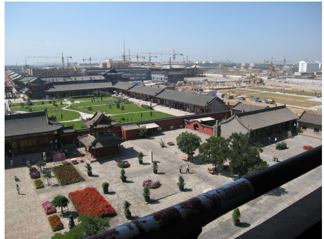
Yingxian Wooden Pagoda #3878 Built 1056 AD, View
