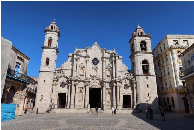
Cathedral #0014 Completed 1777 - Coral Stone
