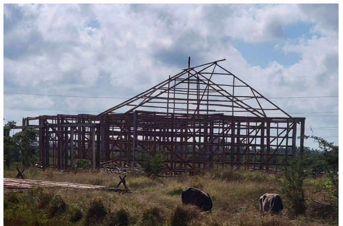
Hurricane Ian #1020 Destroyed Barn
