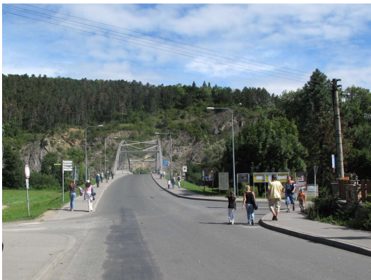
Karlstejn img_0725 Berounka River Bridge
