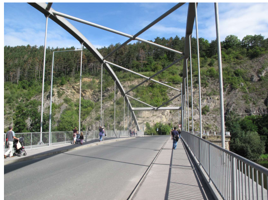
Karlstejn img_0730 Berounka River Bridge
