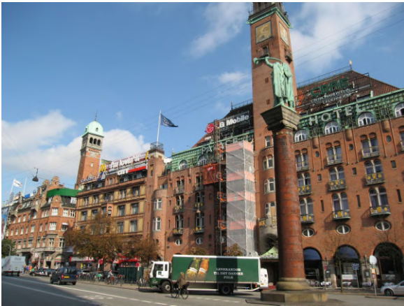
Lur Blower Column #2222
