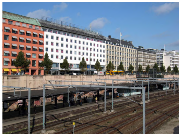
Vesterport #2201 Train Station
