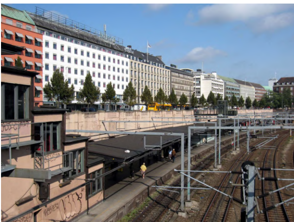
Vesterport #2200 Train Station
