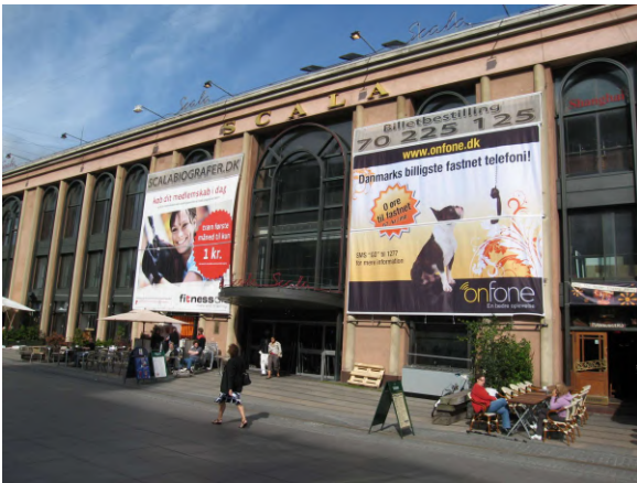
Vesterport #2423 Now Demolished
