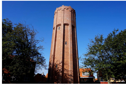
Skagen #2684 Water Tower 1934
