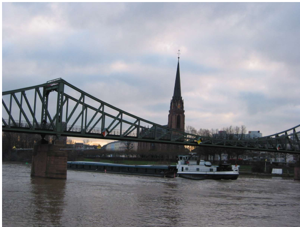
Frankfurt #4606 Iron Bridge
