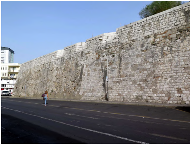
North Bastion #0411 Moorish (Lower) and British (Upper)
