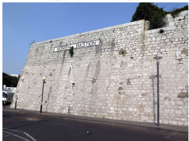
North Bastion #0404 Moorish (Lower) and British (Upper)
