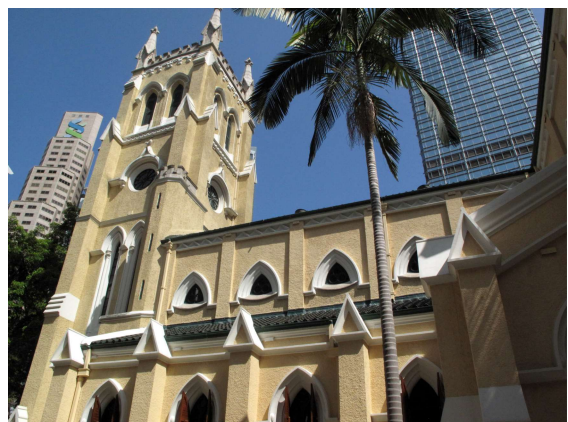
Central #0664 St John's Cathedral (Anglican)
