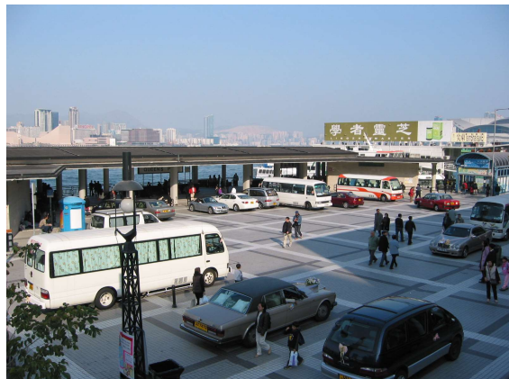
Central #9428 (Former) Queen's Pier
