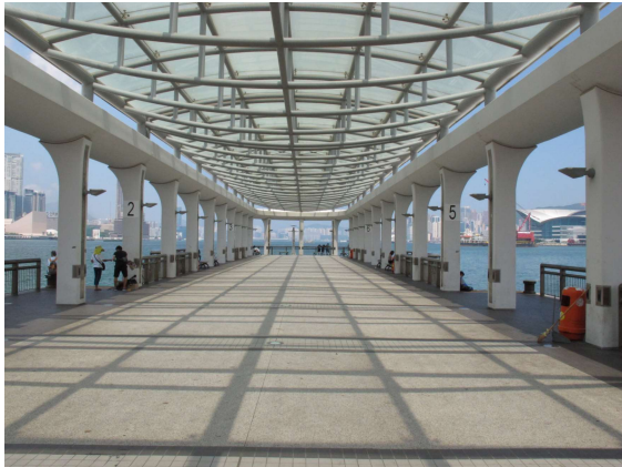
Central #8872 Ferry Pier No 10
