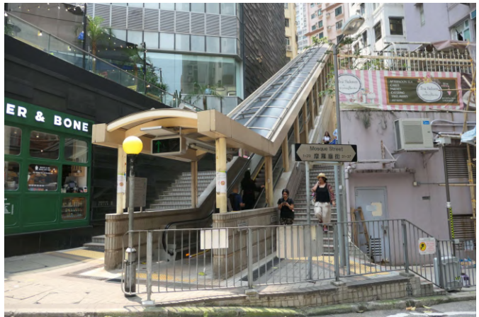
Midlevels Escalator #6079 Mosque St
