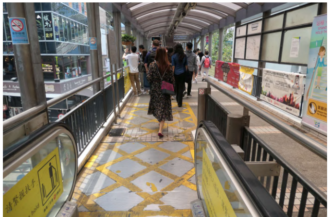
Midlevels Escalator #5953 Connection Between Escalators
