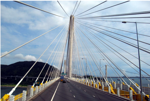
Ting Kau Bridge
