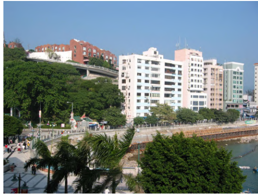
Stanley #4425 Waterfront Rebuilding
