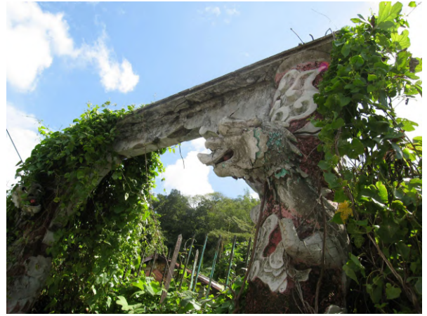
Tai O #0604 Crumbling Old Gateway
