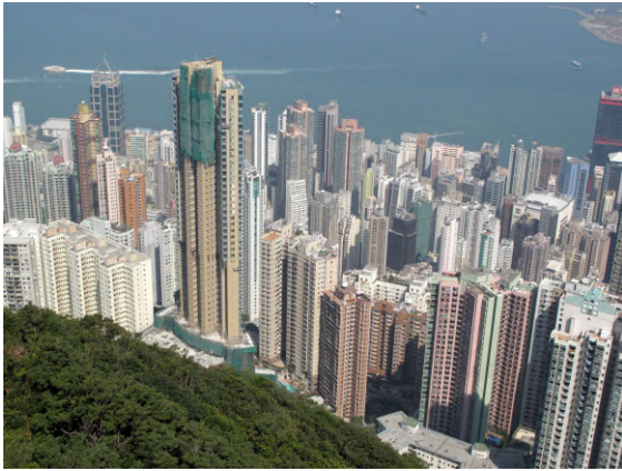
Peak #1351 View of Central - Scaffolding
