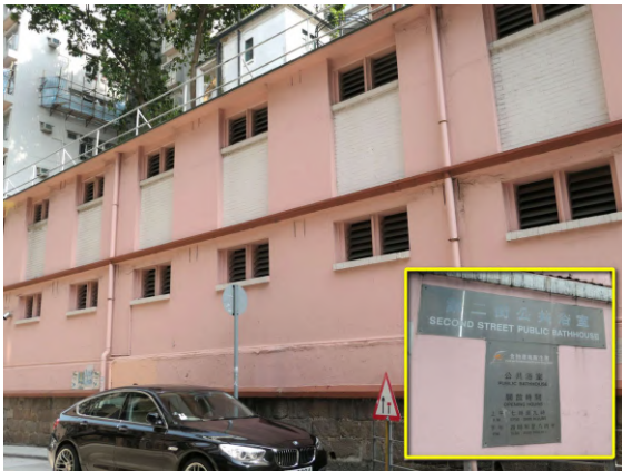
Public Bathhouse - Free Hot Showers Since 1925
