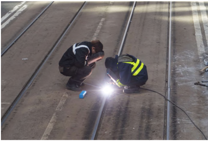
Tram #4708 Tram Track Welding
