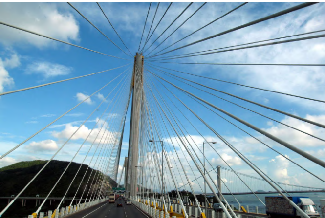
Ting Kau Bridge #9167
