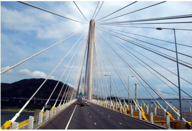
Ting Kau Bridge #2330
