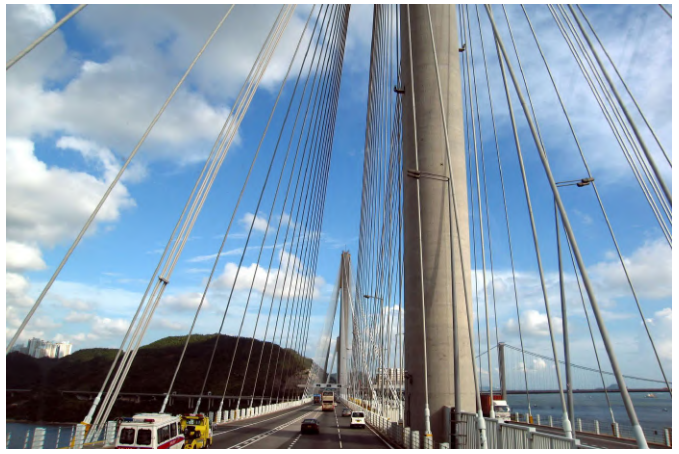
Ting Kau Bridge #9165
