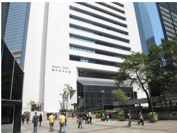
Wan Chai #1261 Wanchai Court Building
