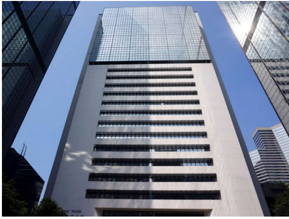
Wan Chai #1264 Wanchai Court Building
