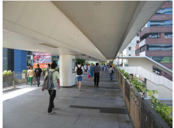
Wan Chai #1745 Footbridge
