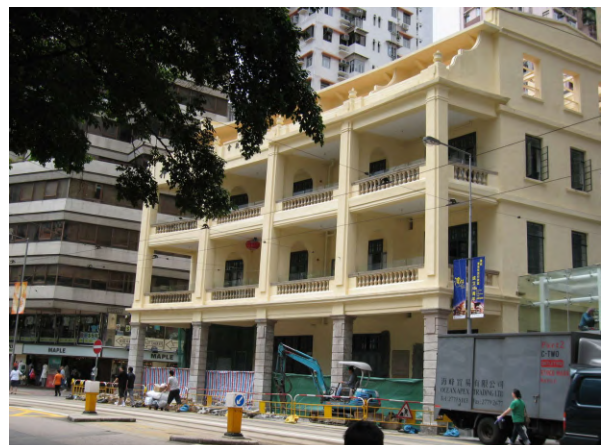
Wan Chai #2387 The Pawn - Renovations Not Finished
