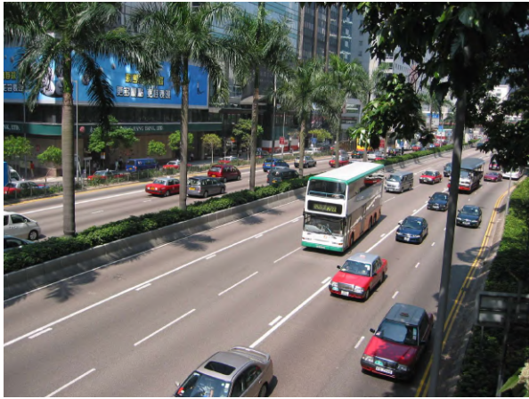
Wan Chai #1486 Gloucester Road
