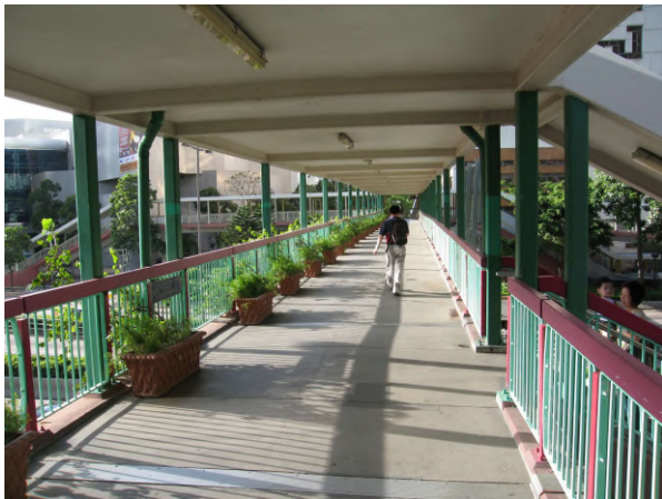
Wan Chai #9172 Footbridge
