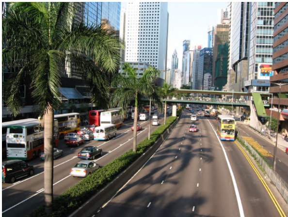
Wan Chai #1492 Gloucester Road
