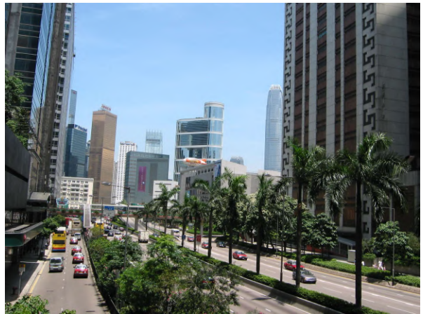
Wan Chai #1468 Gloucester Road
