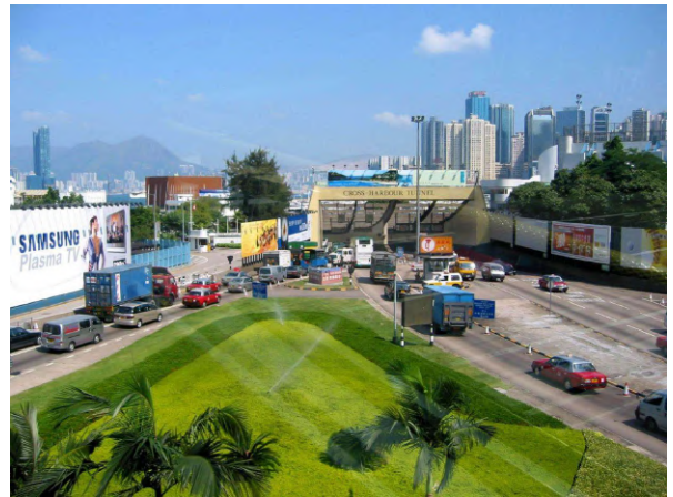
Wan Chai #1822 Cross Harbour Tunnel Wan Chai Entrance
