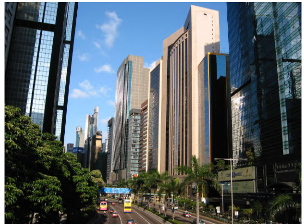
Wan Chai #1495 Gloucester Road
