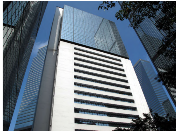
Wan Chai #1259 Wanchai Court Building
