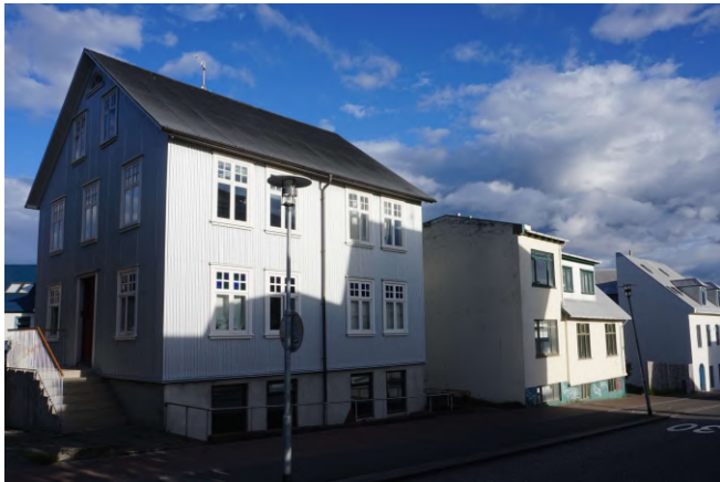
DSCO4059 Reykjavik Corrugated Steel
