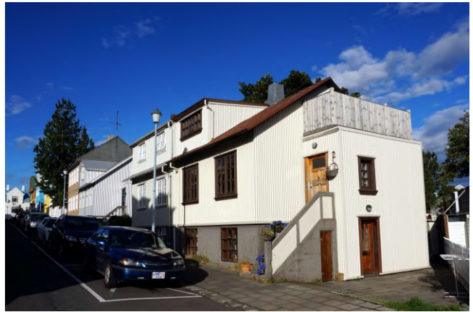
DSCO4071 Reykjavik Corrugated Steel
