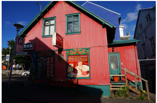
DSCO4064 Reykjavik Corrugated Steel
