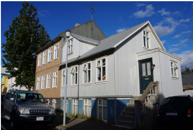
DSCO4073 Reykjavik Corrugated Steel
