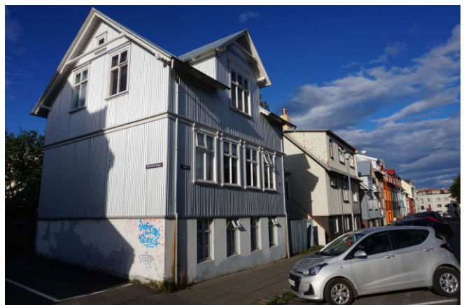
DSCO4066 Reykjavik Corrugated Steel
