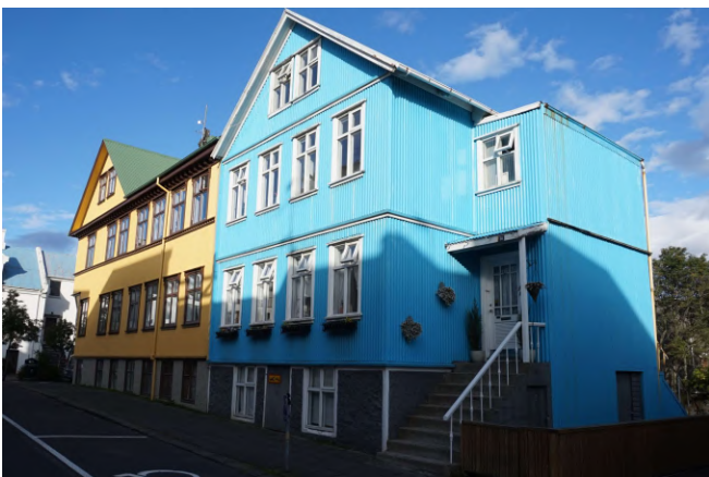
DSCO4076 Reykjavik Corrugated Steel
