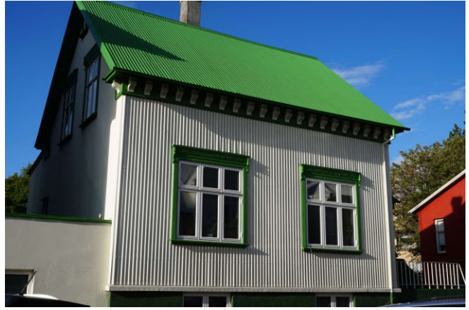
DSCO4068 Reykjavik Corrugated Steel
