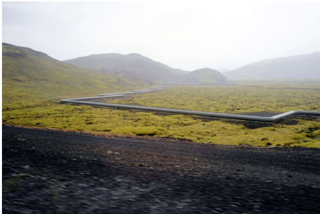
DSCO3641 Geothermal Pipes South Coast
