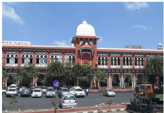
Chennai #7677 Egmore Station
