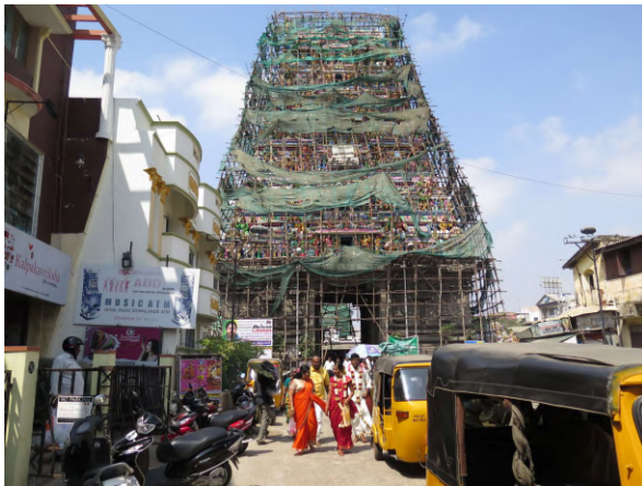
Chennai #5331 Kapaleeswarar Temple Renovations
