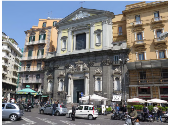
San Ferdinando Church #9733 17th c
