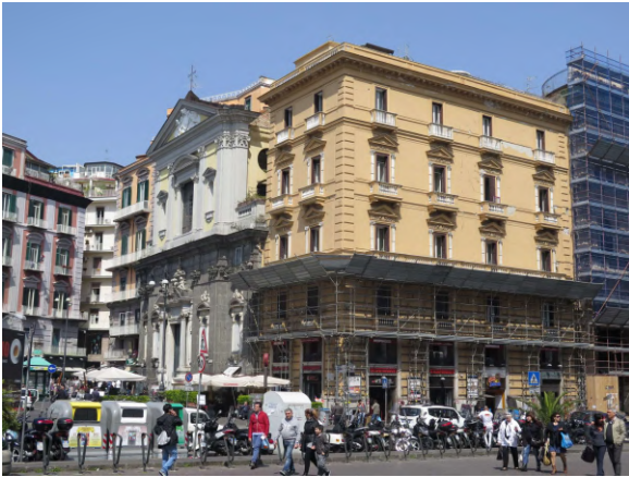
San Ferdinando Church #0941 17th c
