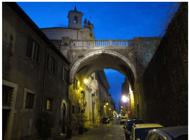
Via Giulia #7206 Michaelangelo's Bridge 1540s
