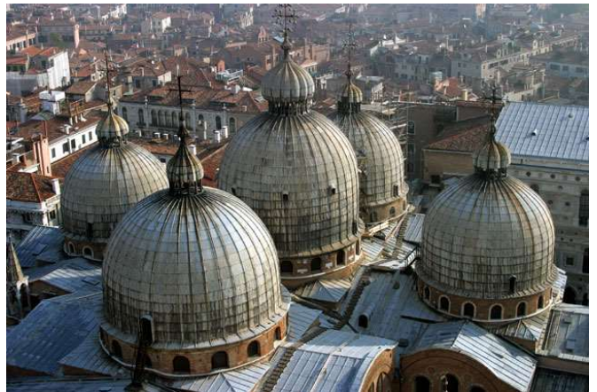
Venice San Marco Roof from Campanile
