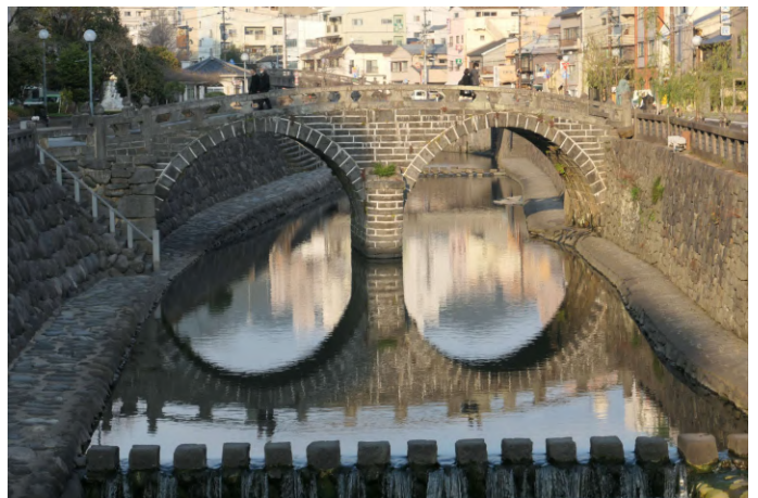
Nakashima River Bridges #3050 Megane Bridge
