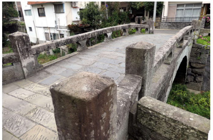
Nakashima River Bridges #2554 Momotani Bridge 1679
