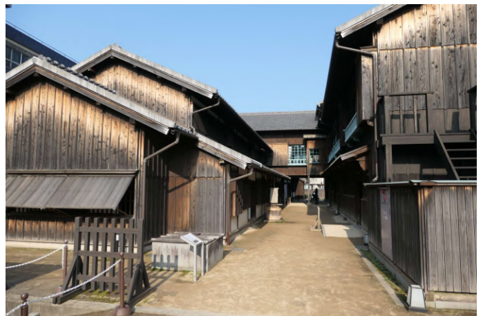
Dejima Island #3549a Dutch Employees Residence Dejima Island
