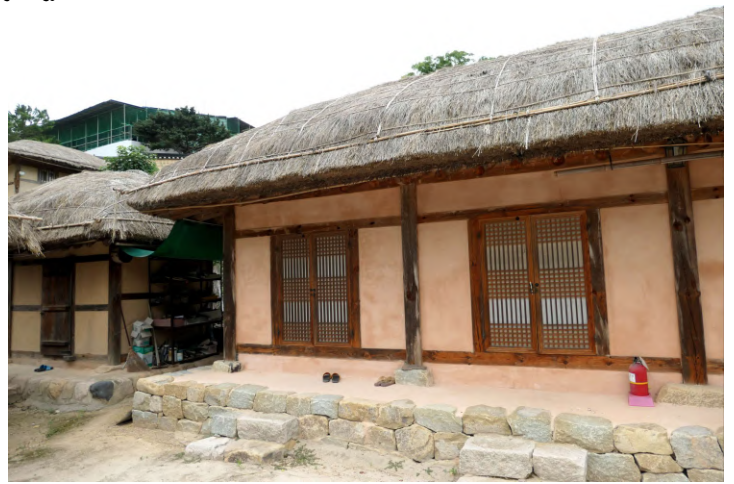
Yangdong Village #8773 Still Occupied
