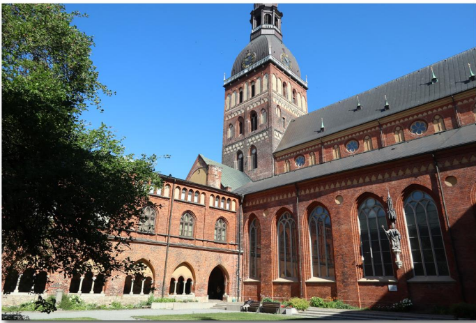
Dom (Cathedral) #9733 Cloister Orig Built 1211
