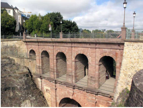
IMG_1305 Castle Bridge 1755 Bock Luxembourg
