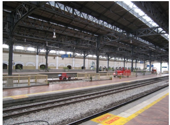
Train Station - Kuala Lumpur #6852
