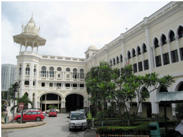
Train Station - Kuala Lumpur #6851
