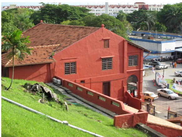
Malaysia Architecture Museum #2015 Historic Govt Building
