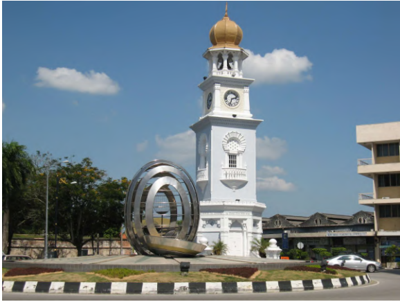
IMG_6058 Queen Victoria Clock Tower 1902
