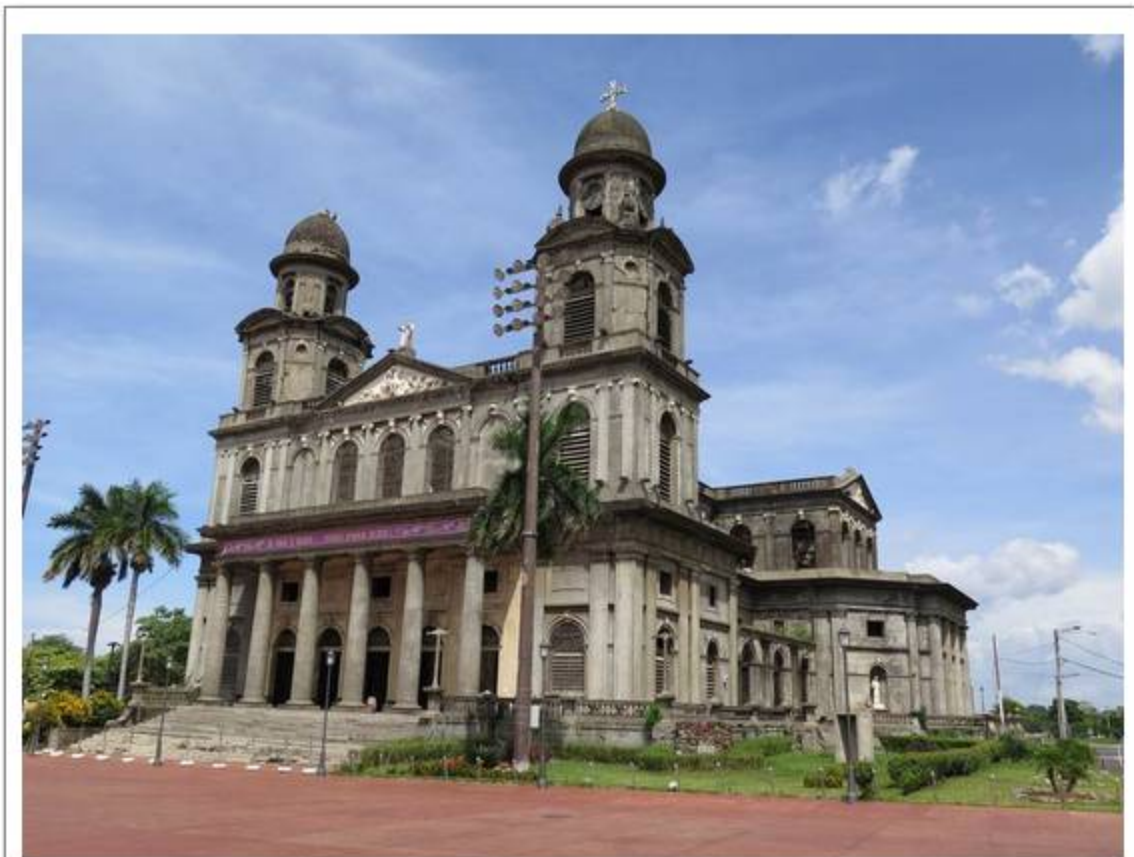
IMG_2687 Santiago of Managua Cathedral 1920 Damaged 1972 Earthquake
