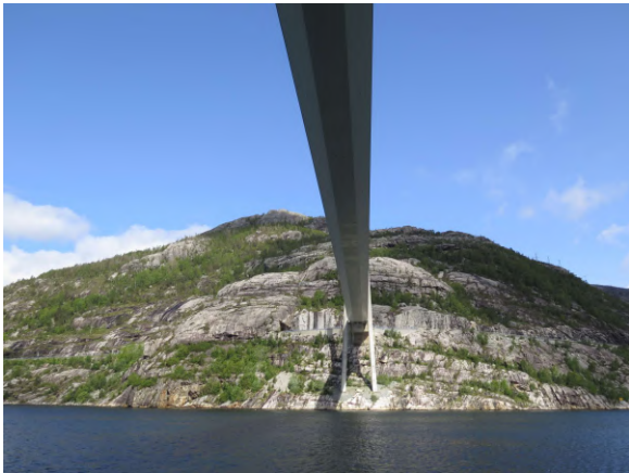
4405 Lysefjord Bridge 2100 Feet
