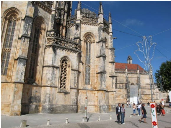
IMG_7583 Batalha Monastery Built 1386-1517
