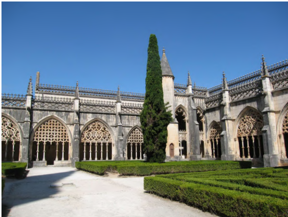
IMG_7631 Batalha Monastery
