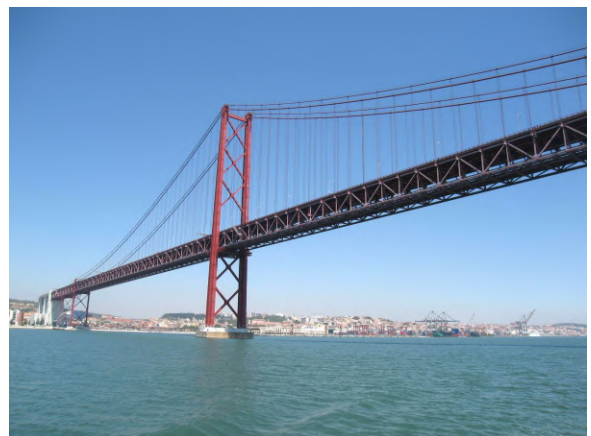
6412 April 25th Bridge Across Tagus River
