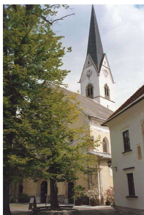
Radovljica 14 St Peter's Church 16th c
