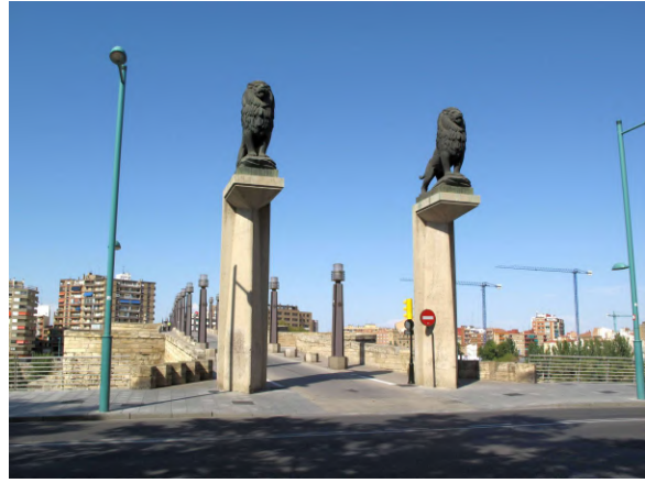
Bridge #6388 15th c Stone Bridge, Ebro River
