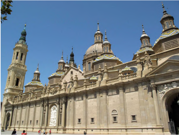
Pilar #6287 Basilica of Our Lady of the Pillar 17th c
