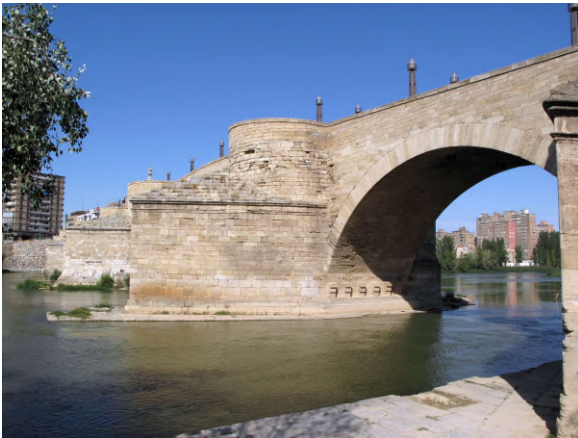
Bridge #6391 15th c Stone Bridge, Ebro River
