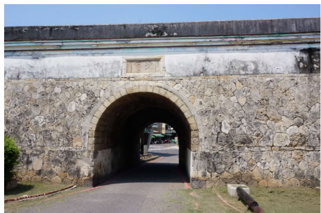
Old City North Gate #0690 1825
