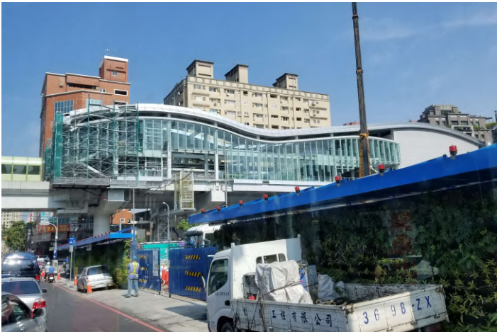
Misc #9291 Metro Under Construction
