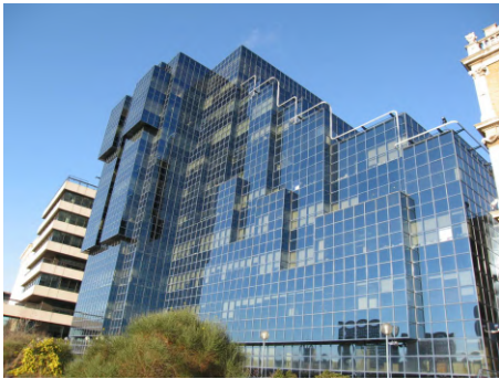
City #1108 Northern and Shell Bldg
