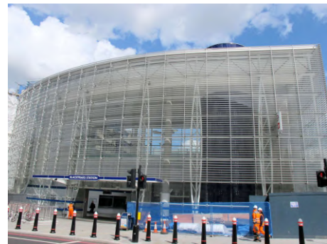
Blackfriars #1754 New Rail Station
