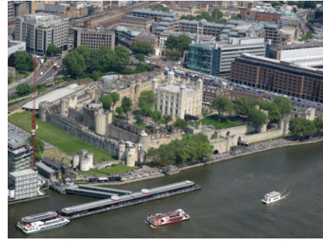
Shard #0180 View of Tower of London
