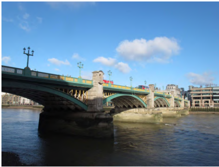
Southwark Bridge #4247 Opened 1921
