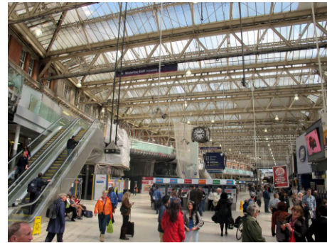
Waterloo #1729 Waterloo Station
