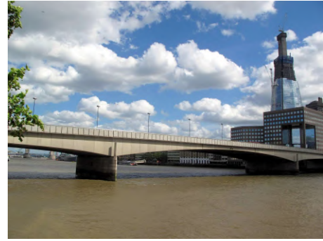
London Bridge #5340 Shard Under Construction
