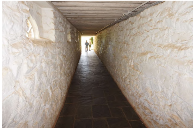
Monticello #7716 Tunnel to Dining Room
