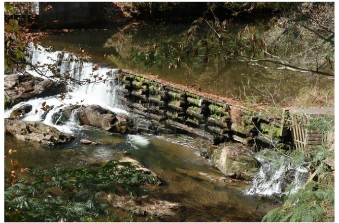
Helen to Sautee Trail IMG_6902 Dam at Nora Mills
