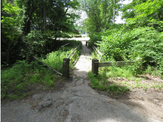
#7646 Blacksmith Rd Bridge
