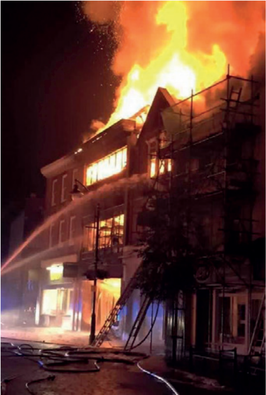
Figure 3.5: A town centre shop fire spreading vertically, horizontally and laterally to involve surrounding buildings. Image courtesy of Russ Talliss via Kent-online
