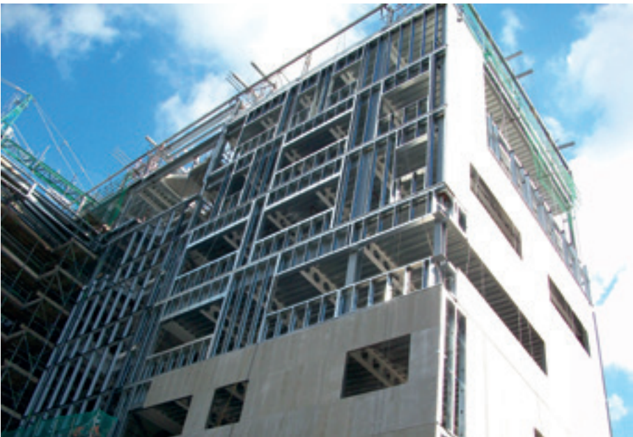
Figure 2.7: Lightweight steel construction is becoming popular in residential dwellings Image courtesy of Graham Couchman Steel Construction Info (SCI)
