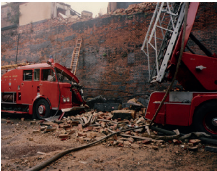
Figures 15.1; 15.2 and 15.3: The corner of masonry warehouse wall collapse that killed a London firefighter in 1978 and critically injured several other firefighters. Photos courtesy Paul Wood
