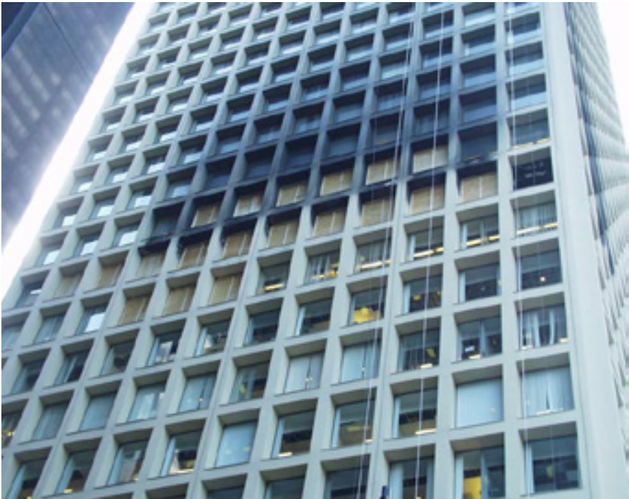
Figure 6.1: The high-rise fire at 69 West Washington (CCAB) Chicago in 2003. Image courtesy of National Institute of Standards and Technology (NIST)
